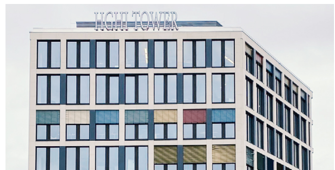
HGHI Tower, CLP Büro Berlin
