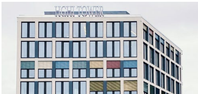
HGHI Tower, CLP Büro Berlin
